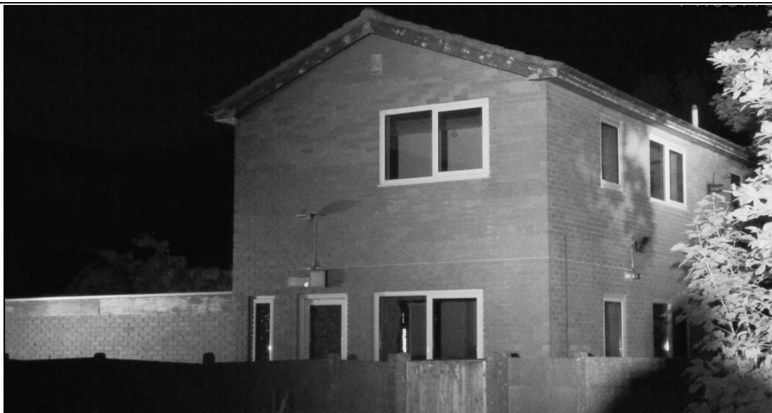
Camera 3 (C3) field of view of Building 2 at the darkest point of the survey, looking at the west gable
