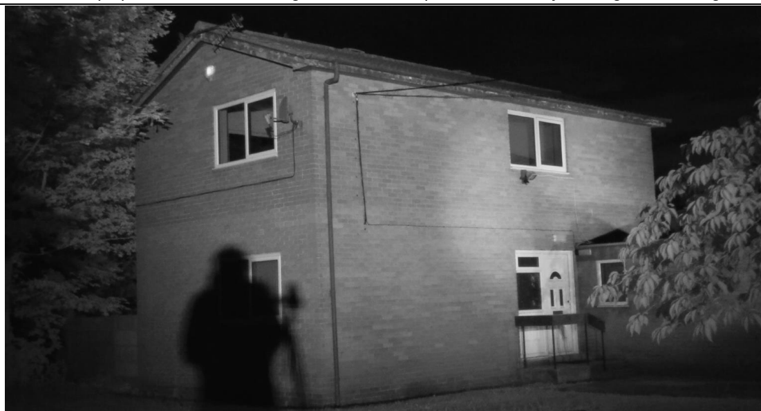
Camera 4 (C4) field of view of Building 2 at the darkest point of the survey, looking at the east elevation
